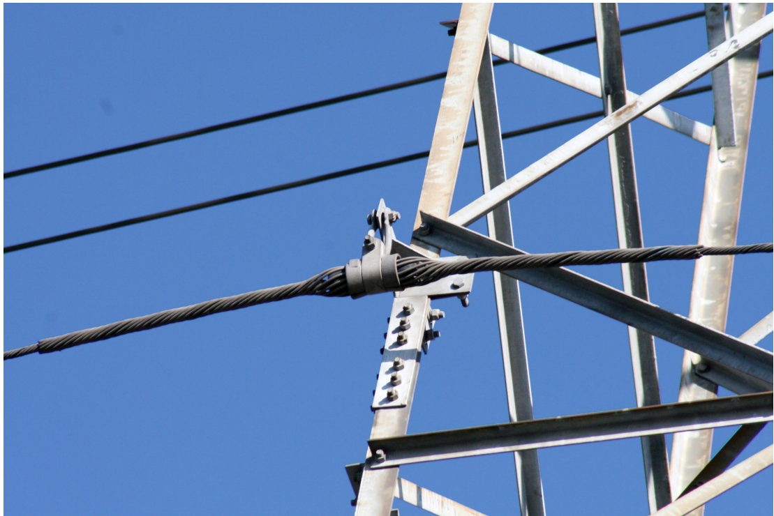
O-ring suspension clamp for ADSS fiber optic cables
